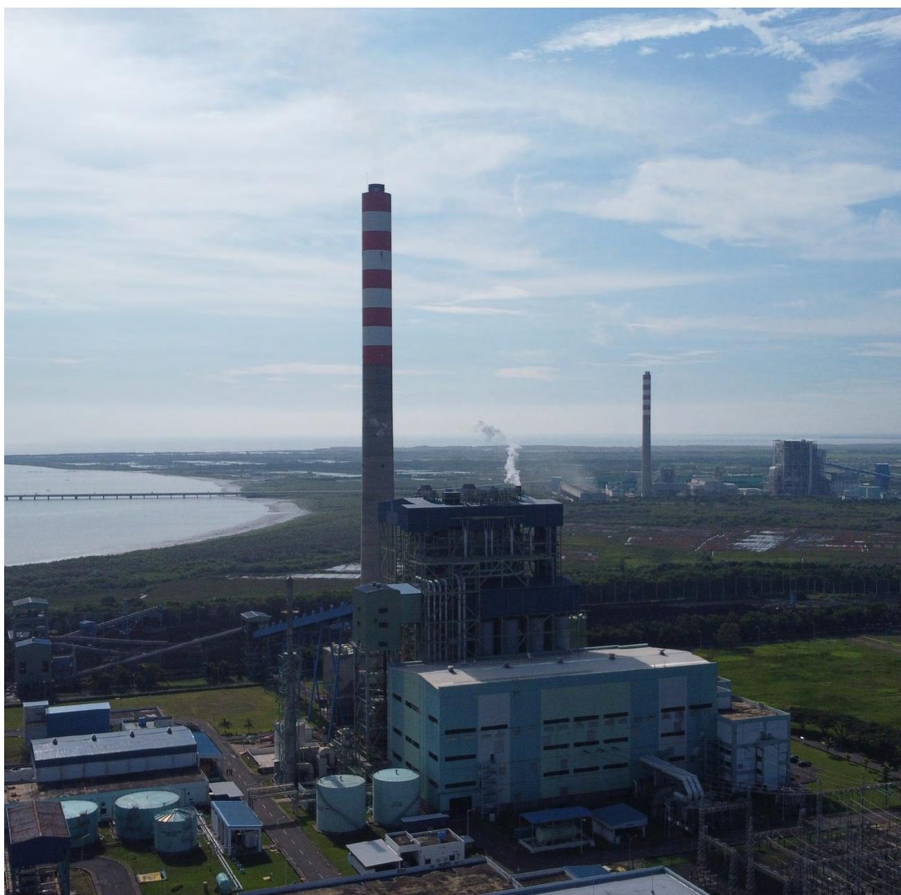
Cirebon 1 and 2 coal-fired power plants, 2023. Photo credit: WALHI West Java.
