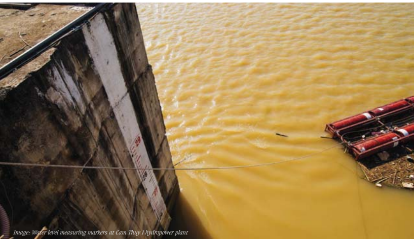
Image: Water level measuring markers at Cam Thuy 1 hydropower plant
