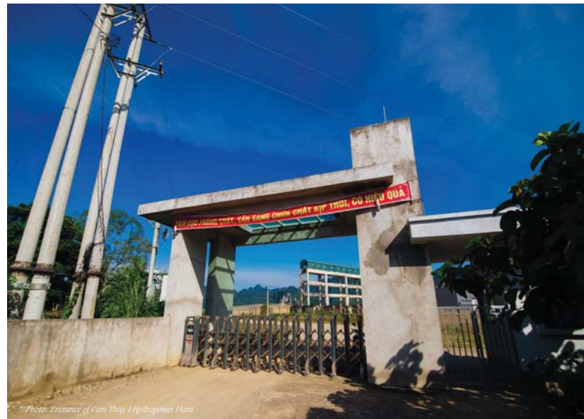
69 Photo: Entrance of Cam Thuy I Hydropower Plant
