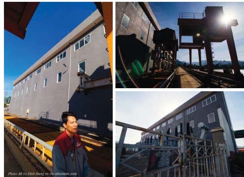
Photo: Mr Le Dinh Hung on the abutment zone
