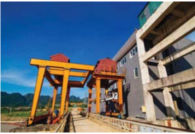
Photo: Cam Thuy Hydropower Plant
