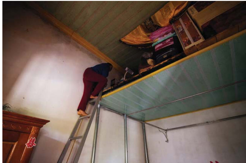
Photo: Miss Mai Thi Hien's attic, for flood prevention
