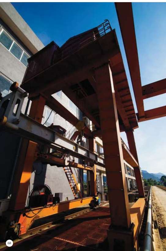
Inlet gate of Cam Thuy I Hydropower Plant
